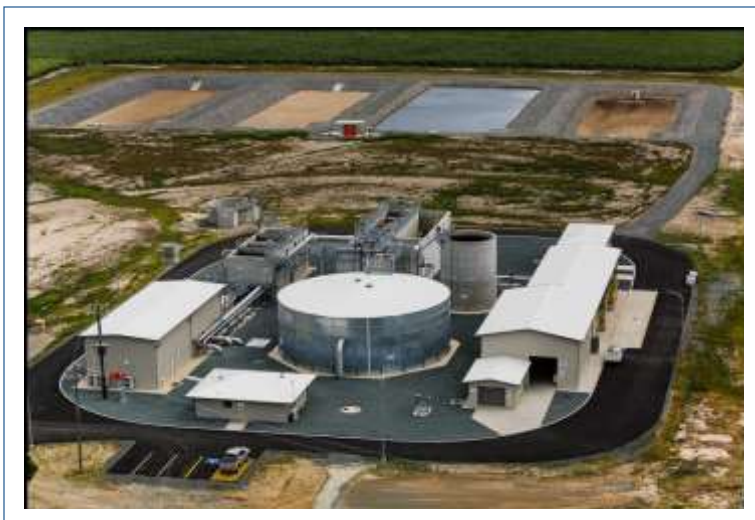
Bowen Water Treatment Plant
