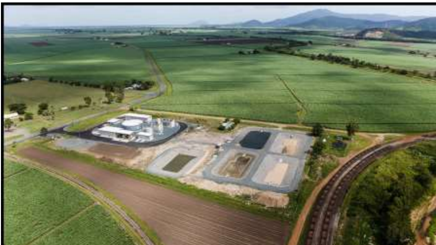
Proserpine Water Treatment Plant
