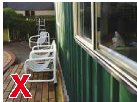
Windows that provide easy access to the pool area must be fixed permanently closed.
