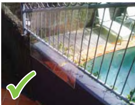
A flat polycarbonate sheet can be used to shield a climbable object.
